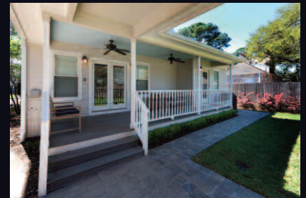
Home Addition Under $150,000 GREYMARK CONSTRUCTION COMPANY
