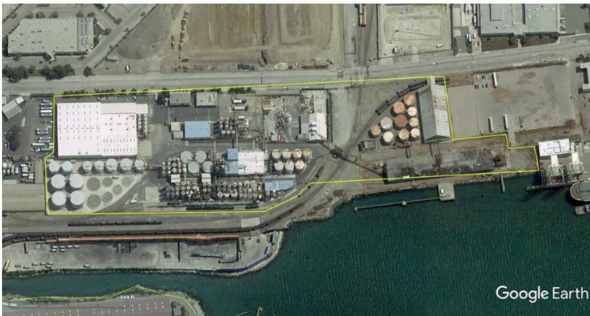
Exhibit 205: Port of Richmond Terminal 2
