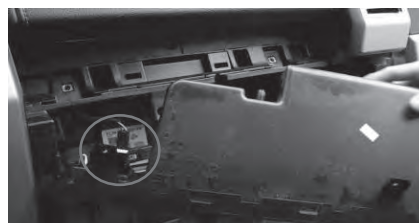
Drop unit out and disconnect wiring at back of unit
