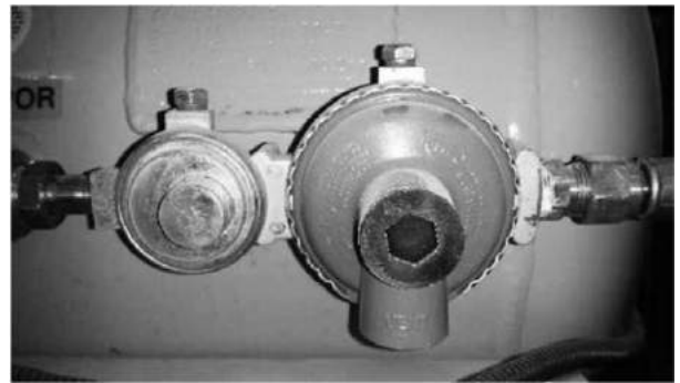
Figure 2-4 LP Gas Regulator
