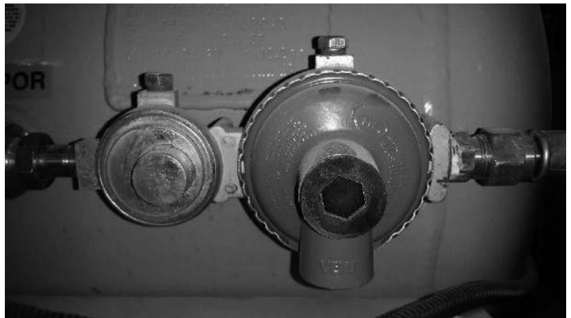
Figure 4-2: LP Gas Regulator
