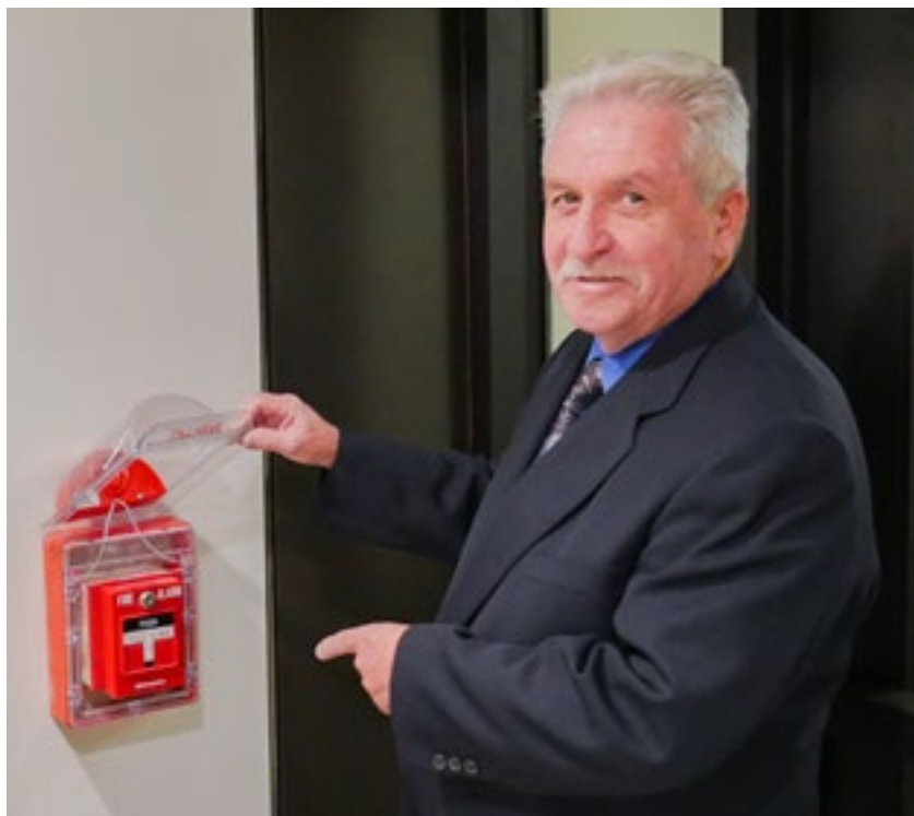
Fire Marshal John Maule inspects the fire alarm box for proper functional operation.
