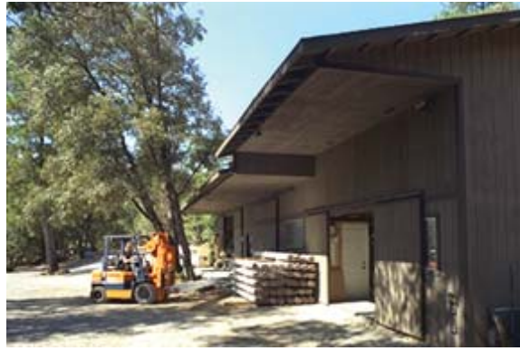
Modern, automated manufacturing & assembly facility
