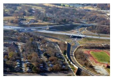
The Salem Creek Connector project is a new, 1.1-mile, four-lane median divided road with sidewalk and greenway connections connecting Martin Luther King Jr. Drive to Rams Drive at the Piedmont Triad Research Park in Winston-Salem. It opened in April 2018. This new road adds nine bridges over parts of Salem Creek and U.S. 52. Also, a new interchange was built at U.S. 52. The current interchange at Rams Drive will be removed.
