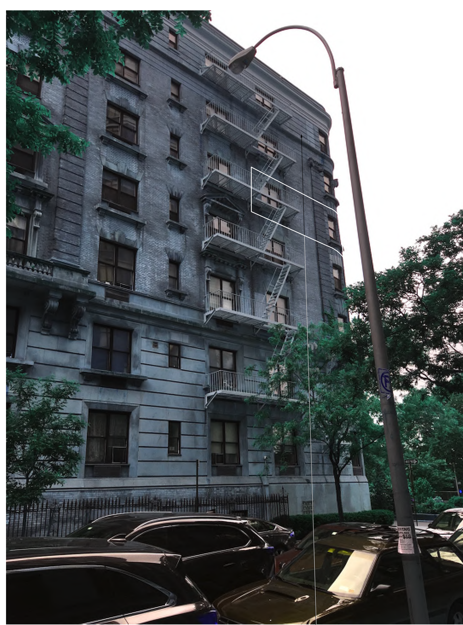
WINDOWS TO BE REPLACED, APT. 508/509
