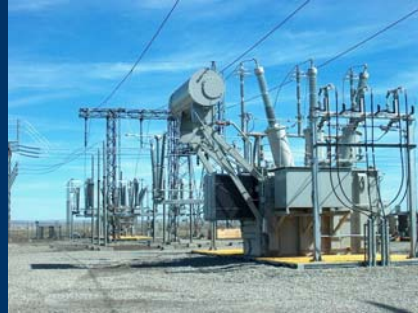
230-13.8 kV Transformer
