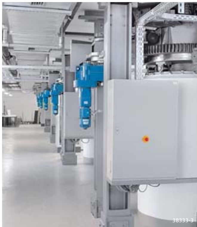
Rotating glass doors at Autostadt in Wolfsburg: The doors are opened and closed smoothly and gently by Demag offset gear motors with a particularly high gear ratio
