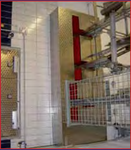
Three continuous conveyor
