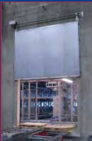
Two continuous chain conveyors
