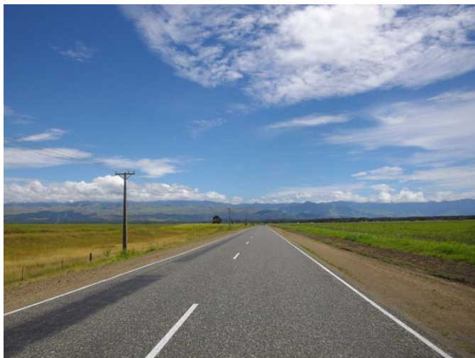
Parallel lines run through the Markham Valley, Morobe.
