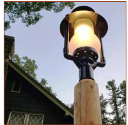
Exterior lighting inspired by Stickley's original lampposts for Craftsman Farms were installed across the property in 2018.
