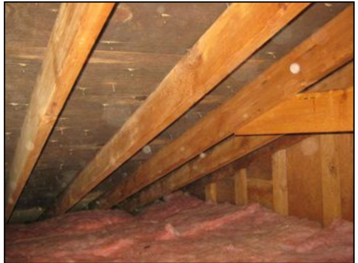
mold on roof sheathing in attic
