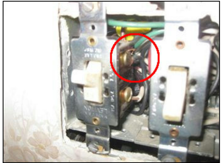
stranded wire entering switch box from basement
