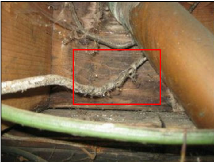
damaged wire in rear band joist
