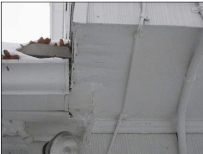
minor damage to lower rear soffit
