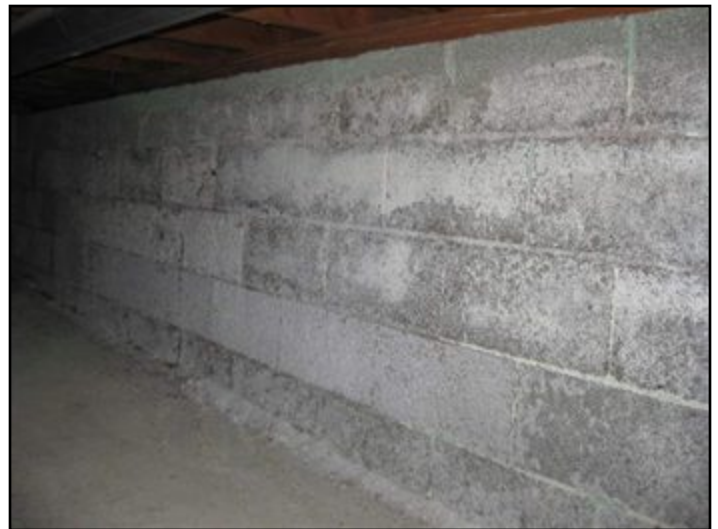
stains on crawl space walls
