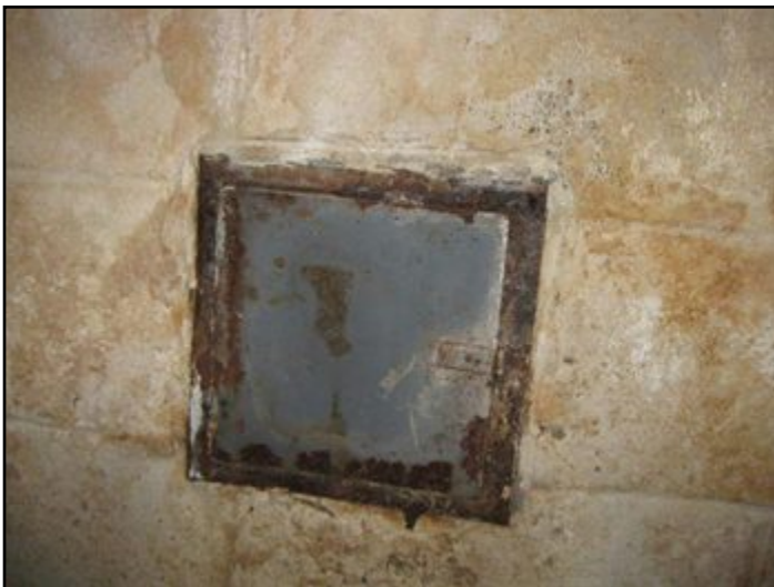
rusted out ash dump door in crawl space
