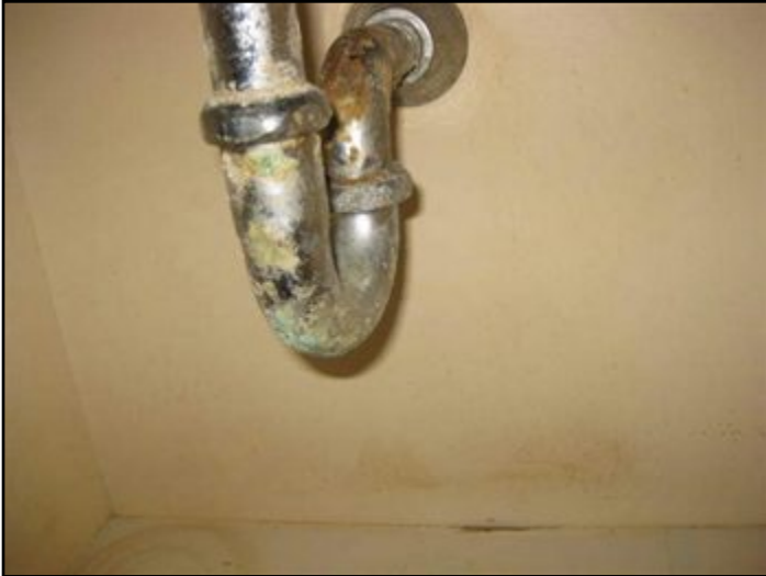
corroded sink trap
