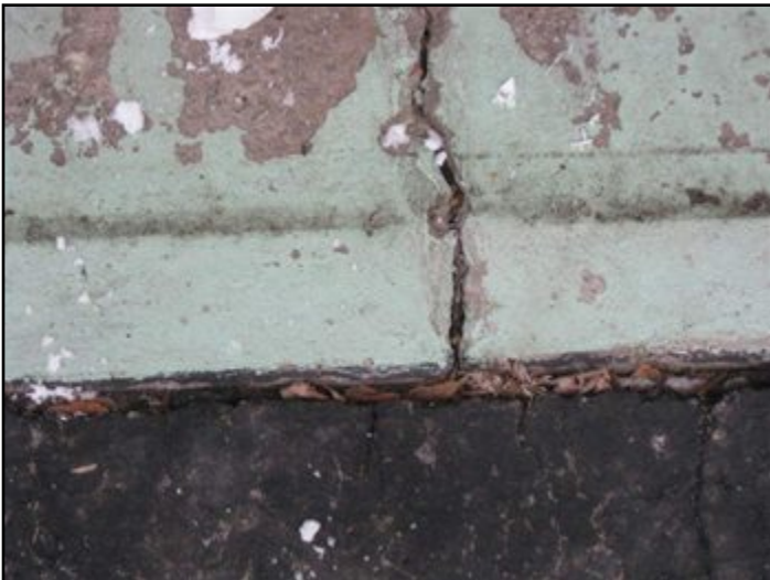
gap between driveway and garage
