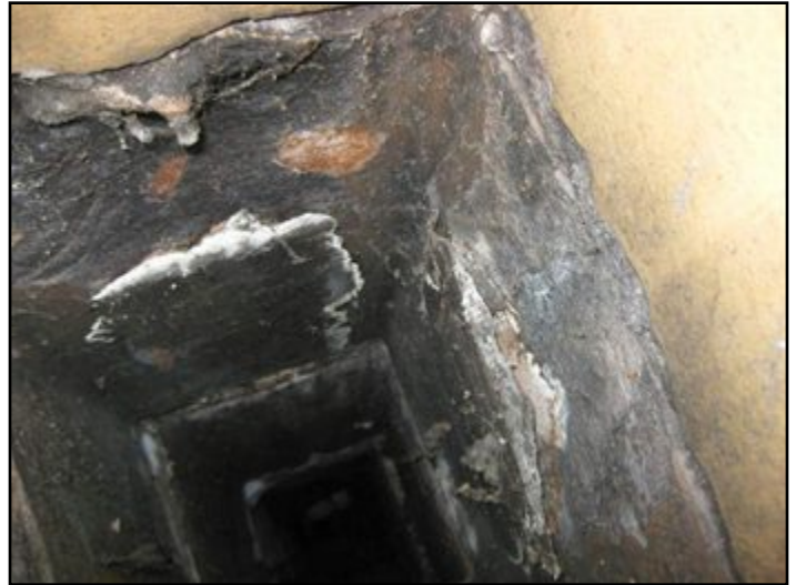
deteriorated, spalled flue tiles
