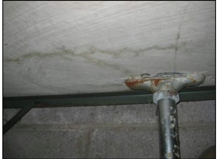
cracks in bottom of laundry tub
