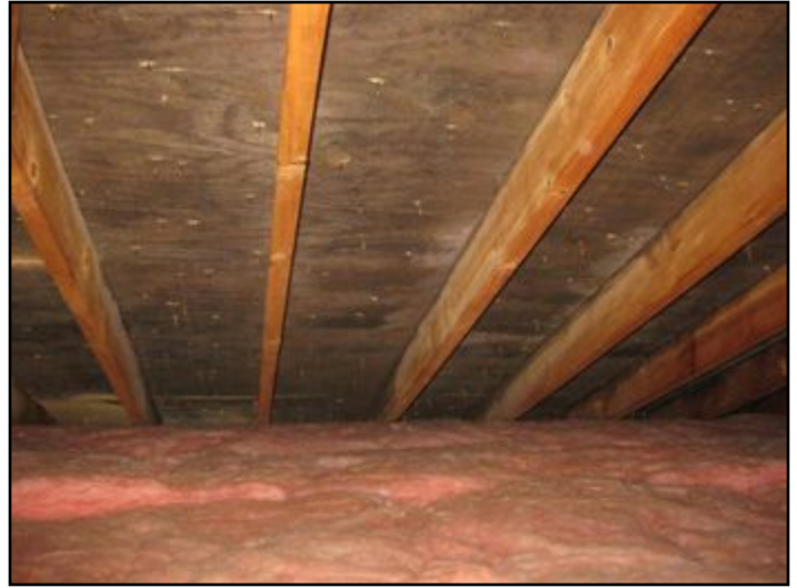
mold on roof sheathing in attic
