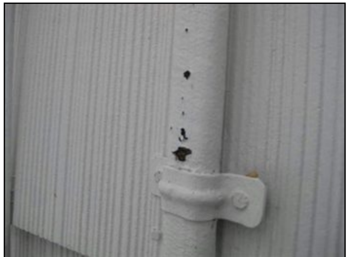
damaged insulation on riser cable
