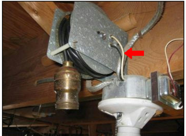
inappropriate wiring at light fixture
