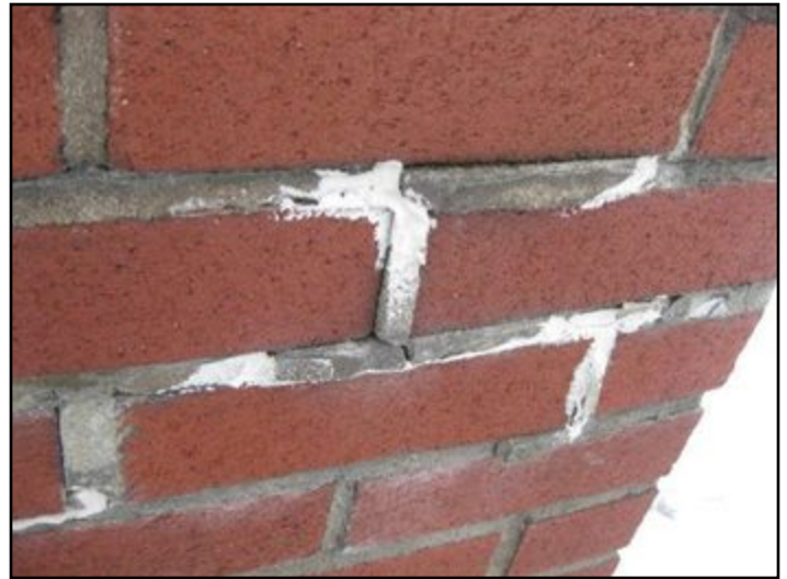
loose mortar, previous repairs
