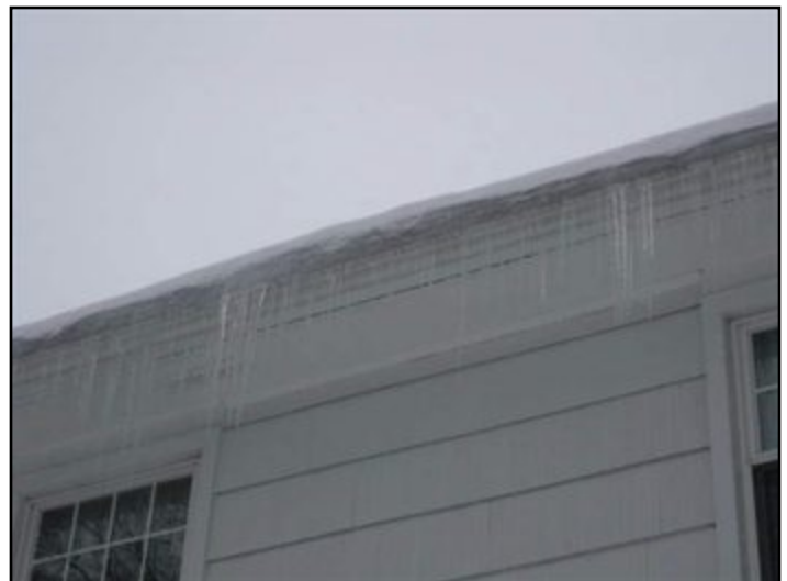
ice buildup in gutters
