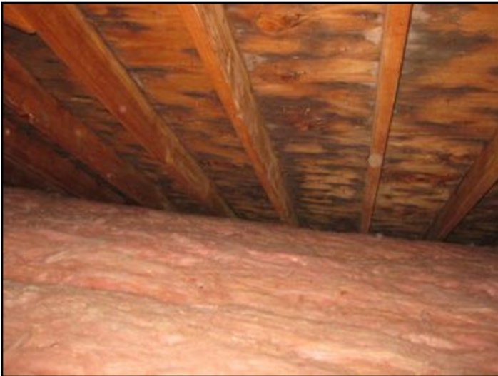
mold on roof sheathing in attic
