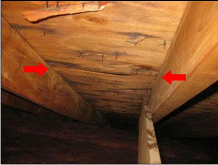
buckled plywood sheathing in attic
