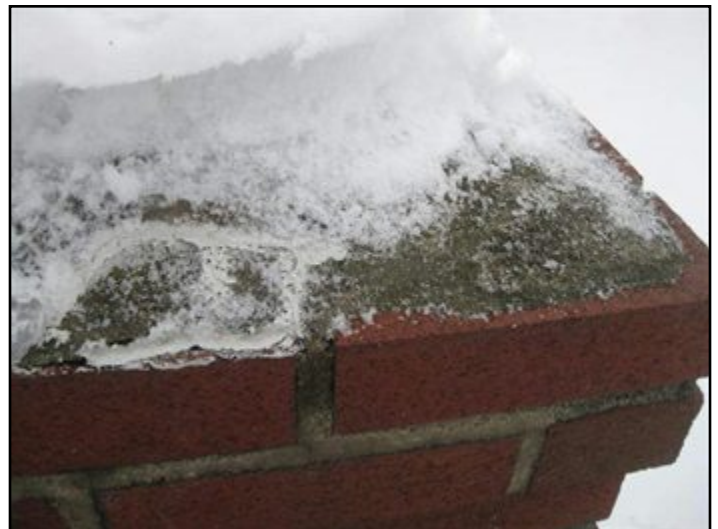
previous repairs, no drip edge (thin at edge)
