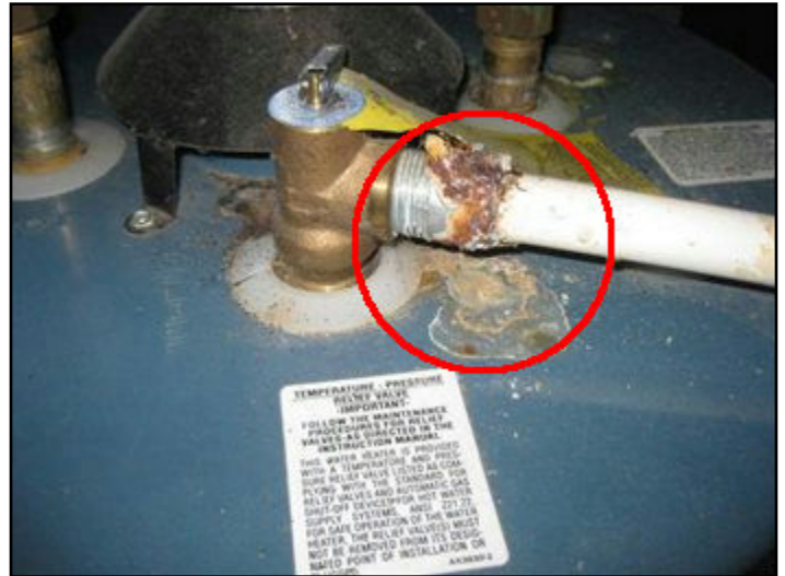
dripping pressure relief valve (PRV)
