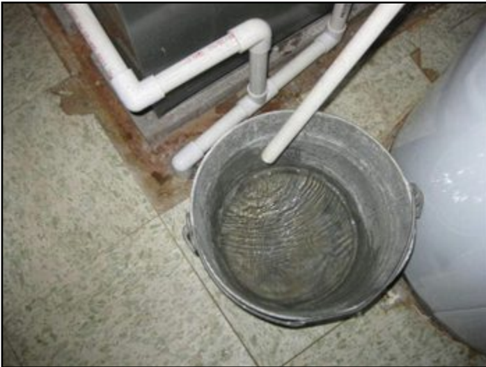
bucket of water from PRV
