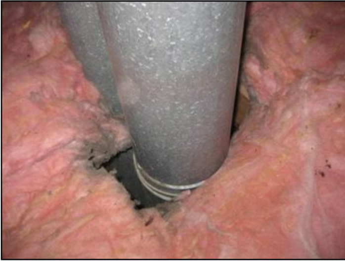
gaps and voids around heating vent pipes
