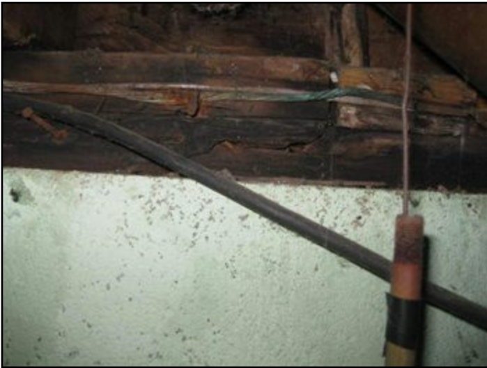
rotted sill plate on rear basement wall
