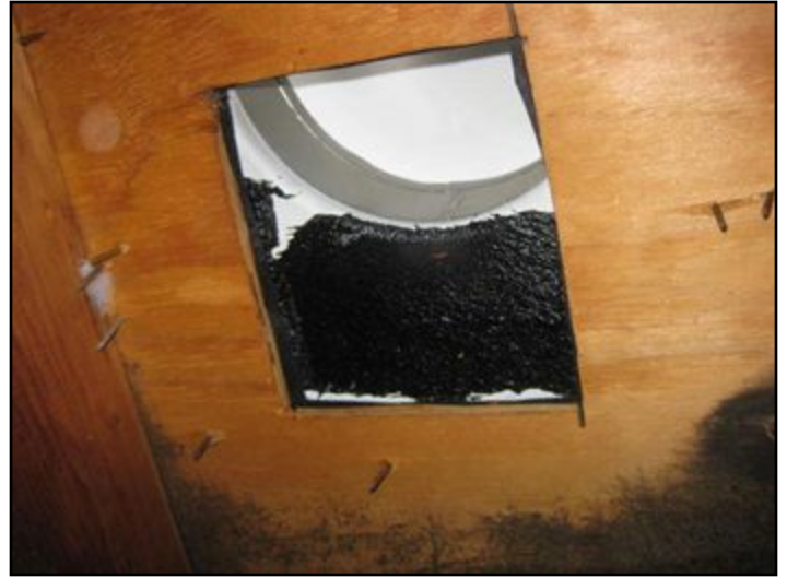
obstructed roof vent
