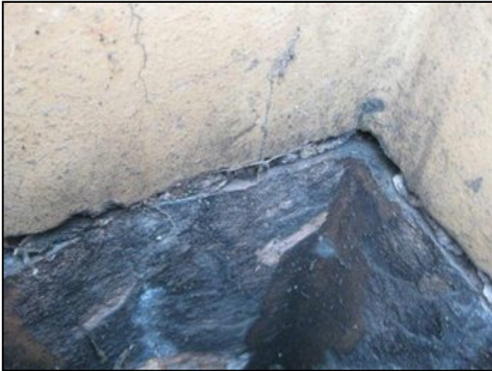
spalled tile, voids between tiles
