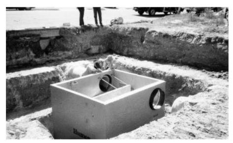
Figure 34.B1 Humeguard<sup>™</sup> Trap
