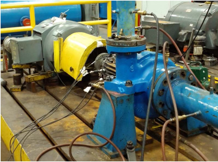
Figure 9a: Pump installed in the test loop
