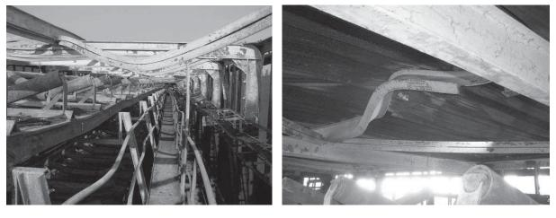
Figure 4.1.5. Deformed upper stiffening truss.
