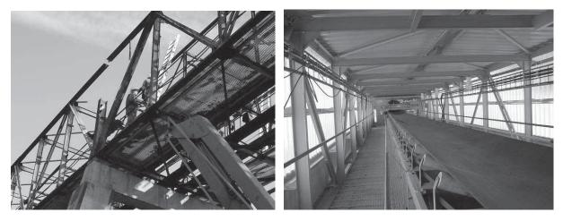
Figure 4.1.7. Replacing of the end frame.
