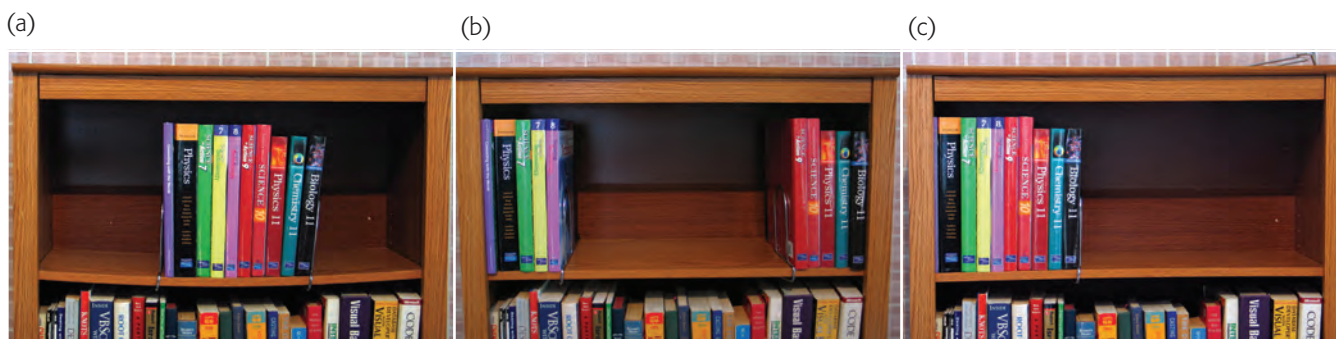
Figure 4.19 When the books are placed in the middle of the shelf (a), the shelf may sag from the unsupported dynamic load. If you place the books nearer the supports ((b) and (c)), the shelf does not sag.
