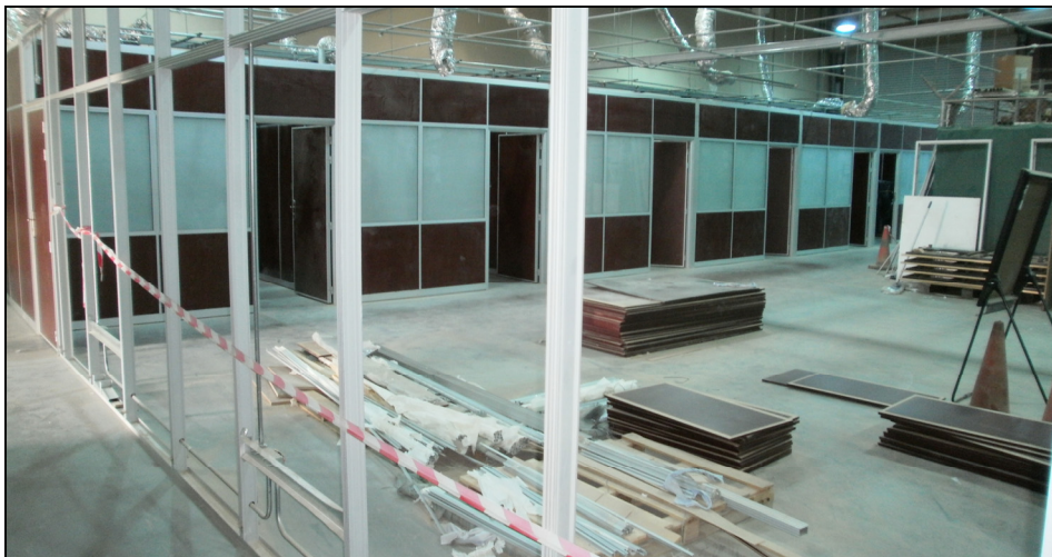
Office space and living quarters are being added in Kuwait.
