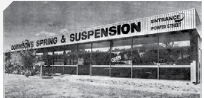
1991 - Dobinsons Spring & Suspension moves to it's current Head Office location
