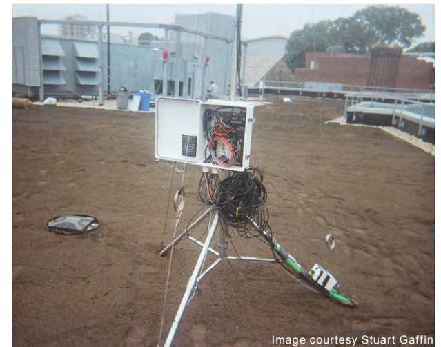
Data logger during the installation of an experimental green roof
