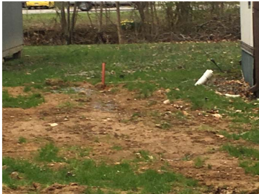
Sewer line installed, not yet connected to mobile home.
