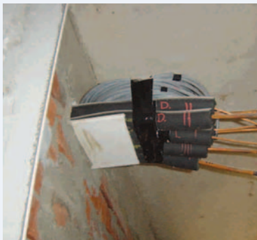
1. Routing of pipes in the trunking box
