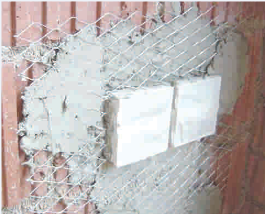
Reinforcement installed around openings for electrical services
