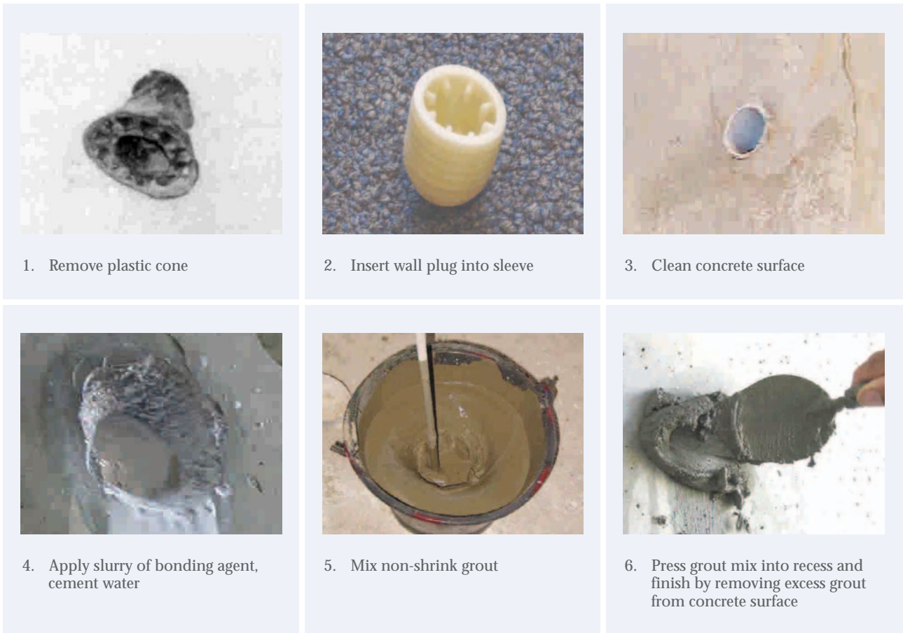
Figure 5.7: Patching of form tie holes
