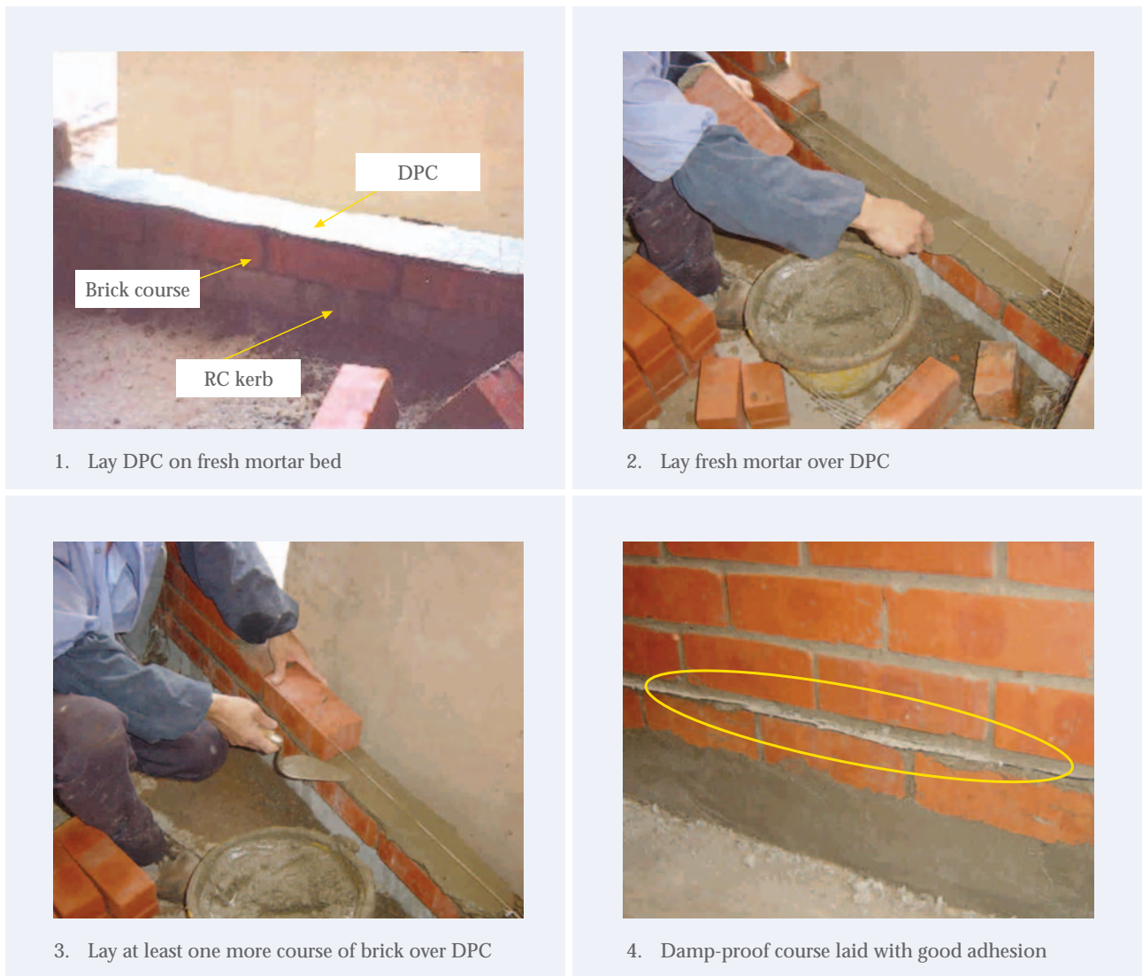
Figure 5.14: Laying damp-proof course (DPC)
