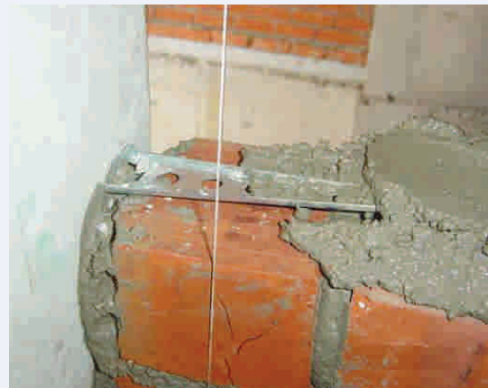
Bonding bars embedded at every 4 th course of brickwork
