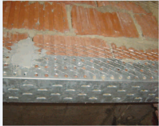
Reinforcement installed around lintel
