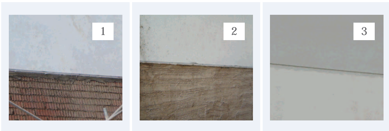
Figure 5.25: Terminating plastering works at groove lines
