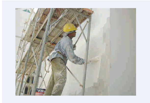
Figure 5.27: Application of sealer prior to painting works
