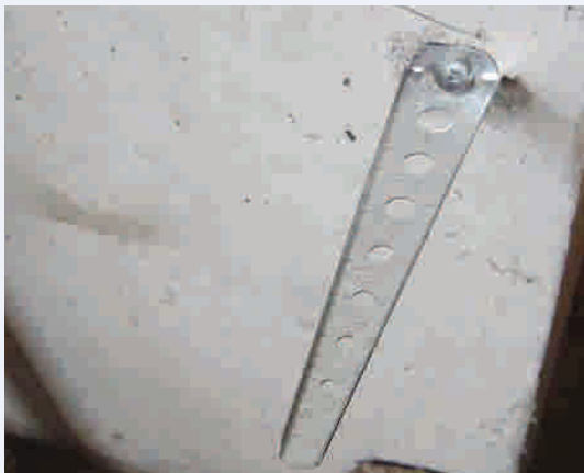
Bonding bars fixed to a concrete column
