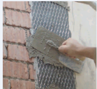
3. Install metal lath at brick-RC joints
