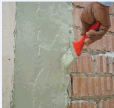
2. Apply waterproofing membrane
