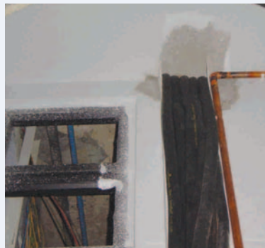
2. Patching surrounding gaps using cement mortar
