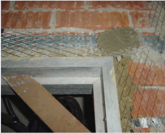
Reinforcement installed around door frame
