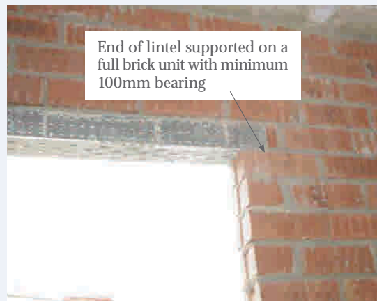
Steel lintel installed at window opening
