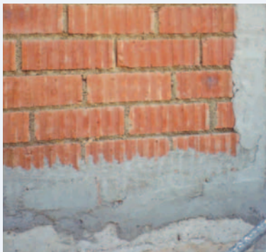
1. Apply render to brick-RC joints
