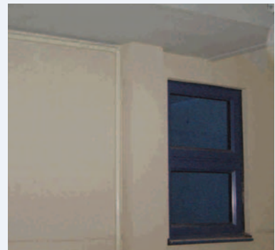
3. Connecting the trunking and finishing with paint
