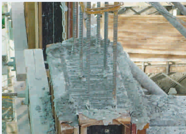
Figure 5.6: Joint surface roughened to improve bonding at RC-RC joint
