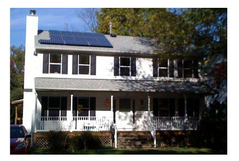
College Park, near Metro Station Installed by StandardSolar.com 10 PV panels (2.15 kW) installed January 25-26, 2011 with battery backup
