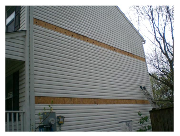
Liquid phenolic foam is pumped between exterior and interior walls and fills all cavities, then turns into solid closed-cell foam. Done by USAinsulation.net
