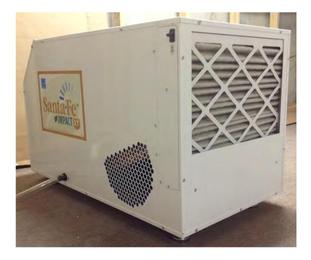
Santa Fe Impact XT, seasonal consumption ~200 kWh, dehumidifies the whole basement and house (using central fan).
