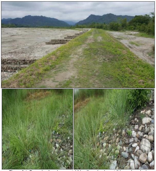
Figure 6-1: Example of environmental friendly embankment (bio-engineering)
