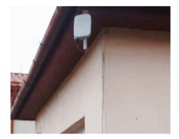
Figure 15 : Outdoor CPE installed in the residence of a friendly user
