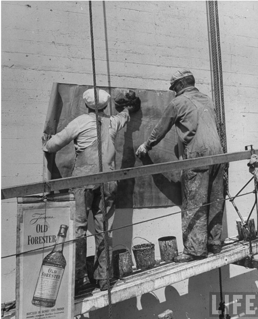
“Pouncing,” a method of patterning a wall with charcoal: 1930’s
