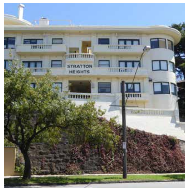
Alexandra Avenue, South Yarra, southern side of river
