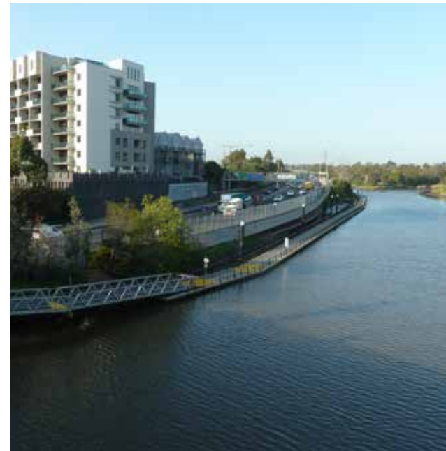
Cremorne, northern river banks, view east from Chapel Street Bridge
