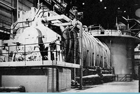
**Reactor & primary** coolant system in a hull section inside a shield water tank
