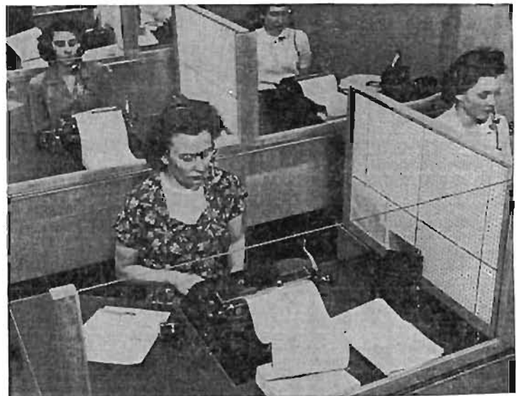
View of new classified phone room, showing individual adtaker's unit, housed in glass and soundproof enclosure, containing specially designed desk, noiseless typewriter with special want ad characters; and lightweight headset.
