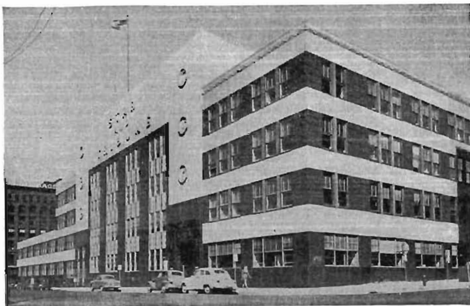
Front view of buff and black Minneapolis Star and Tribune building, covering square block.
