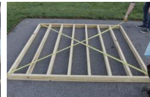
(18) If measurements are not equal, move the ends of the band board left or right, accordingly.
