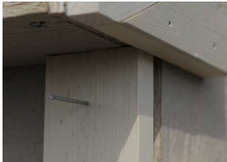
(103) Attach corner trim to side wall, making sure it is flush with the gable wall as shown, using 2” trim nails spaced 8-12” apart, along edge of trim.
