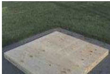
(25) Repeat previous steps for back piece, using an 8" to 12" nail spacing, and ensuring all flooring is either flush or parallel with the floor joists.
