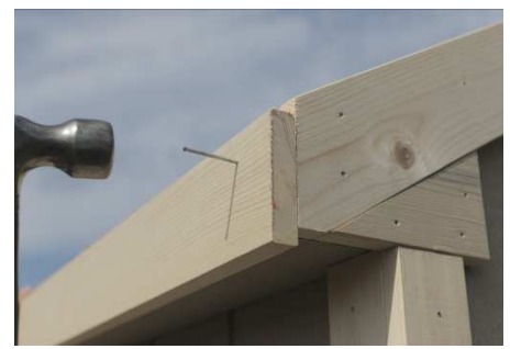
(105) Fasten fascia to rafters, using two 2” trim nails per rafter, and making sure fascia is flush with the top of the rafters, and with the gable fascia.
