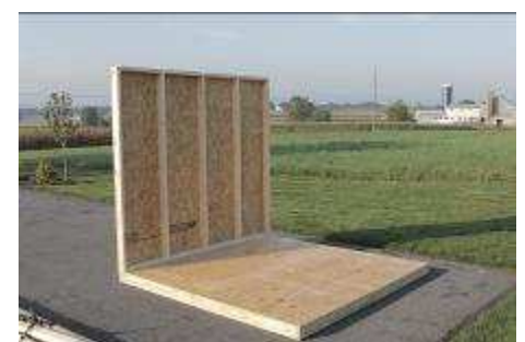
(27) Ready for walls! Refer to next step.
