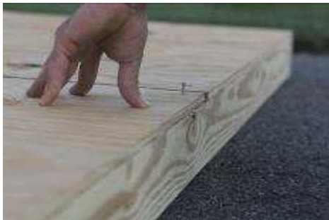
(22) Nail along the gable, making sure flooring is flush with the floor joist. Use an 8" to 12" nail spacing.
