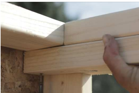
(52) Be sure to fasten the pre-cut blocks on both sides, as done in previous steps for rear gable.
