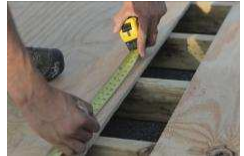
(24) Before you finish attaching the first row flooring to the joist, make marks 12" on center for a guide to adjust the joist when nailing.
