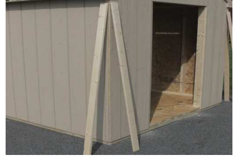
(102) Lay out the corner trim for each corner.
