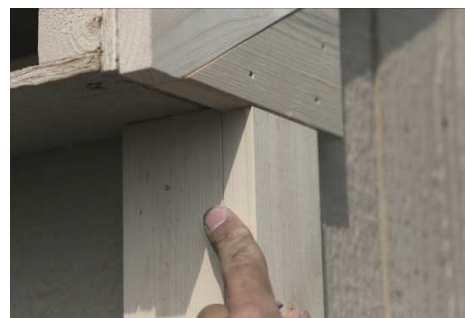
(104) Install the other corner piece as shown. Repeat for rest of corners.
