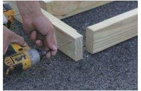
(15) Begin with the end joist, making sure the band board is flush with the joist.
