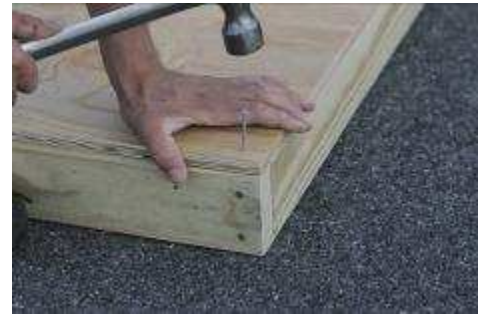
(21) Attach the corner of the flooring, using 2" nails.
