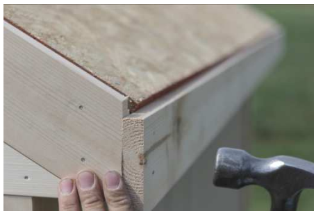
(106) Done! Repeat these steps for the fascia on the back side.
