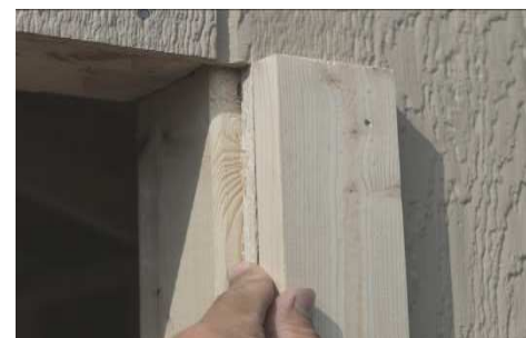
(107) Install right side door trim, staying 1/2” to the right of the door frame, and flush with the top of the door frame.
