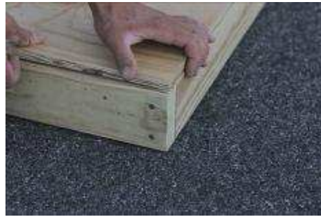
(20) Start on the front right corner with the first piece, making sure flooring is flush with perimeter. NOTE: Both pieces of flooring are 41-7/8"x84"
