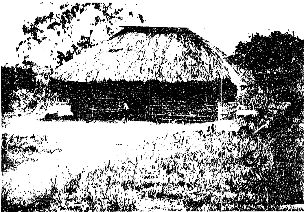
Photograph 10: Typical dwelling in study area—thatch roof, mud-stick construction, cane door, no windows.
