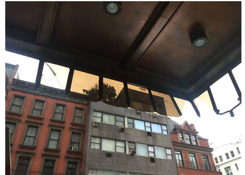
DETERIORATED CONIDITIONS (CURRENT -): FRONT SECTION OF ACRYLIC SKIRT AND SUPPORTING ELEMENTS ARE SEVERELY DAMAGED OR MISSING.
