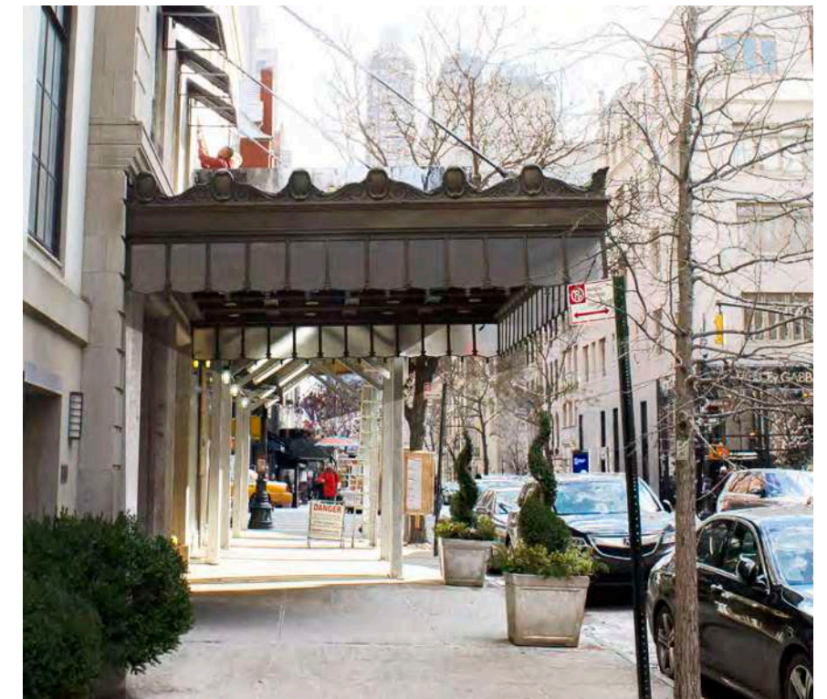
EXISTING MARQUEE ON 69TH STREET (LOOKING EAST) (NO PROPOSED CHANGES)
