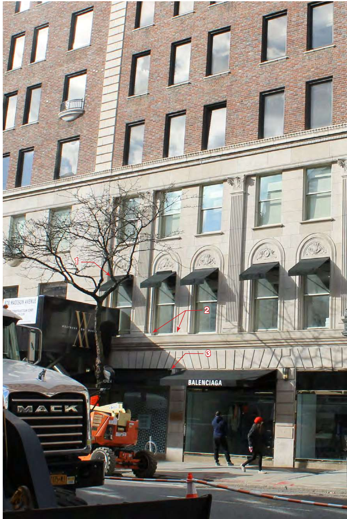
OVERALL MOCK-UP PHOTO: TAKEN ACROSS FROM MADISON AVENUE LOOKING SOUTHWEST
