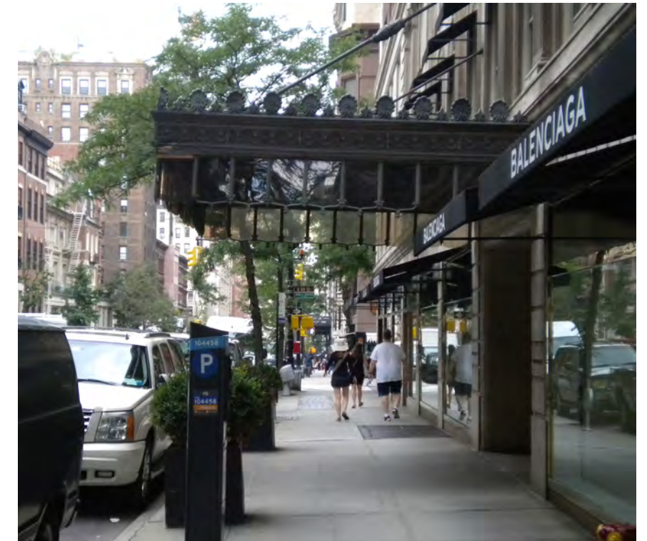
EXISTING MARQUEE ON MADISON AVE (LOOKING SOUTH)
