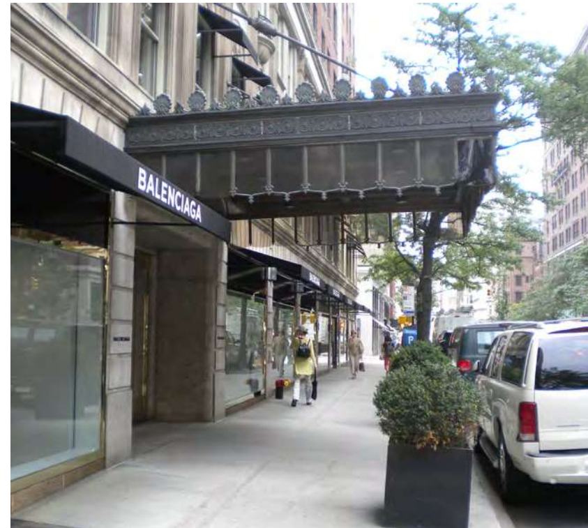
EXISTING MARQUEE ON MADISON AVE (LOOKING NORTH)
