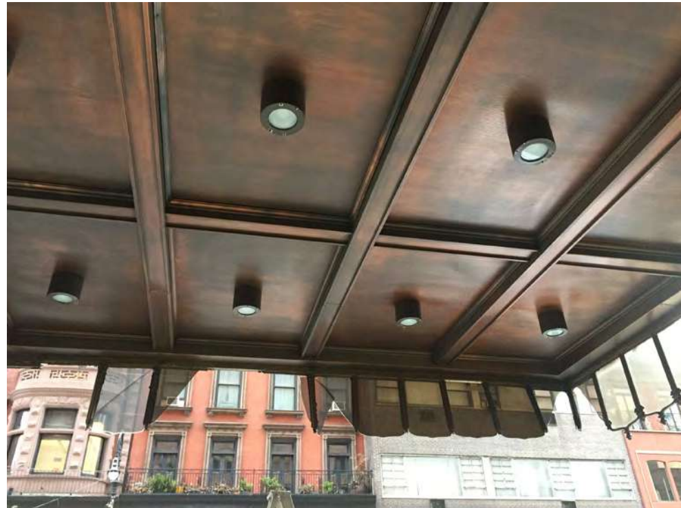
DETERIORATED CONIDITIONS (CURRENT -): FRONT SECTION OF ACRYLIC SKIRT AND SUPPORTING ELEMENTS ARE SEVERELY DAMAGED OR MISSING.
