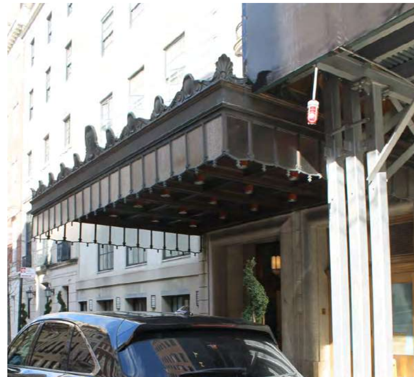
EXISTING MARQUEE ON 69TH STREET (LOOKING WEST) (NO PROPOSED CHANGES)
