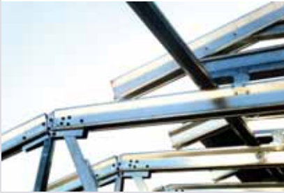
Cap truss installed on top of base truss. Note continuous bracing on top chord of base truss and connection clip.
