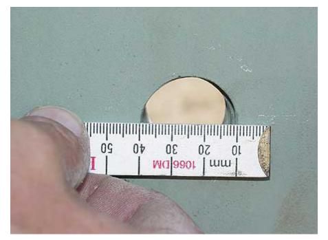
Improperly drilled splice plate
