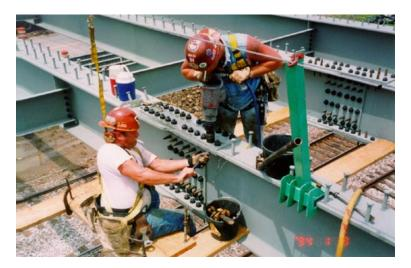
Final Bolting (Note: Drift Pins are still in place.)
