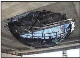
Fall Protection & Debris
