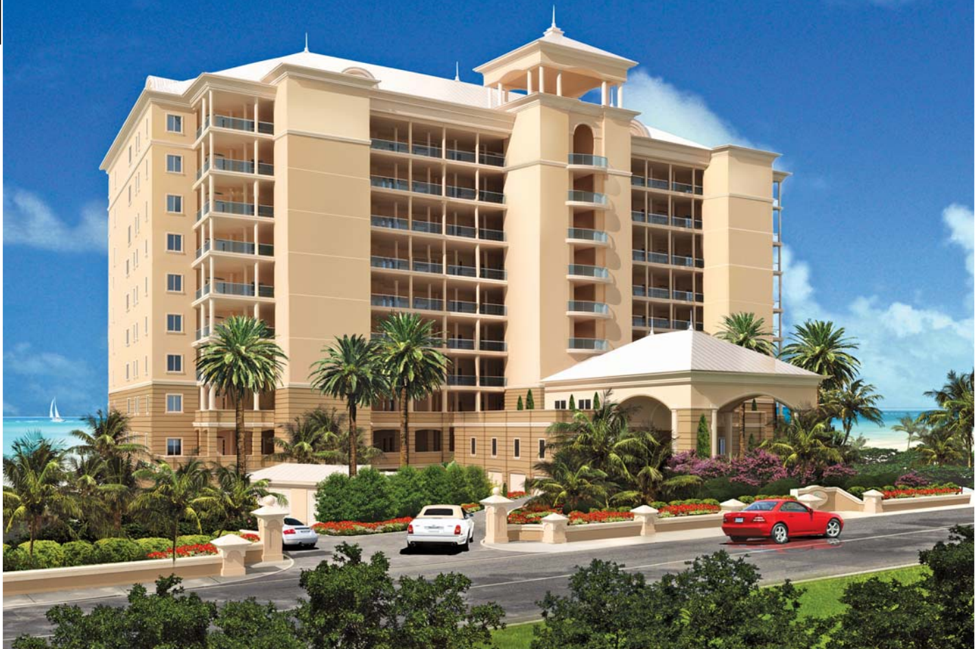
WaterColours, an exclusive enclave of luxury condominiums, under construction on Seven Mile Beach.
