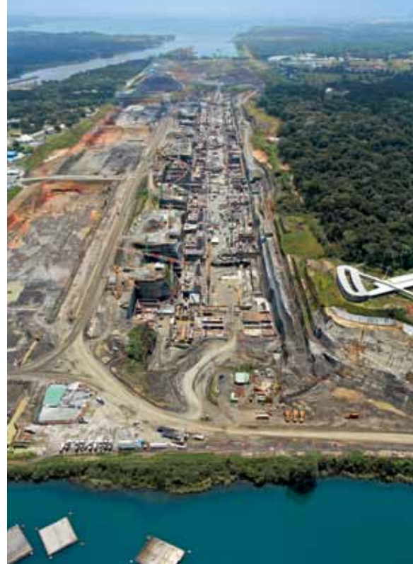
The Gatun lock facility on the Atlantic coast has three chambers positioned one after the other - each of them is 403 m long and 55 m wide. Photo: ACP
