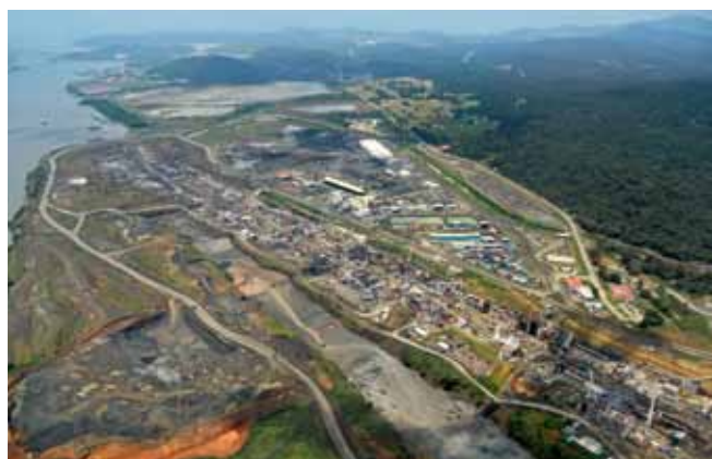
The Miraflores lock system on the Pacific coast is around 1.8 km long and lifts the vessels using three chambers to a height of 26 m above sea level. Photo: ACP
