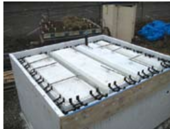
Quad-Lock REM-10 under construction, Quad-Lock REM-10 with green roof layer
