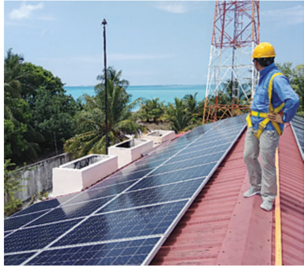
■ POISED = Preparing Outer Islands for Sustainable Energy Development Project. The POISED project has demonstrated significant physical progress with the installation of 1,600 kilowatts-peak (kWp) Solar photovoltaic system in Addu City, S. Hithadhoo at phase 1 (left) and 200 kWp in Kelaa, Haa Ali at phase 2 (right) (photos by Ministry of Environment).
