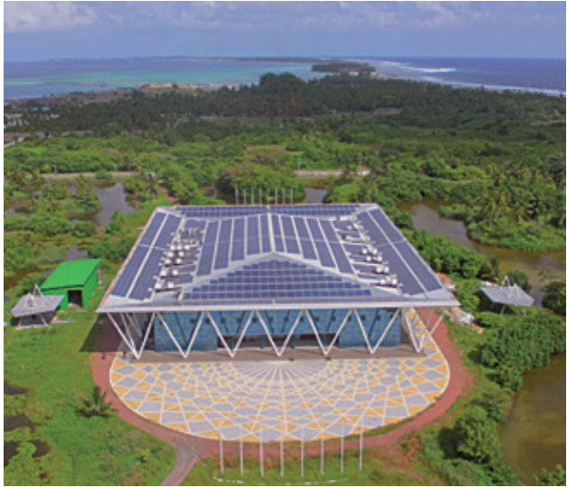
■ POISED = Preparing Outer Islands for Sustainable Energy Development Project. The POISED project has demonstrated significant physical progress with the installation of 1,600 kilowatts-peak (kWp) Solar photovoltaic system in Addu City, S. Hithadhoo at phase 1 (left) and 200 kWp in Kelaa, Haa Ali at phase 2 (right) (photos by Ministry of Environment).
