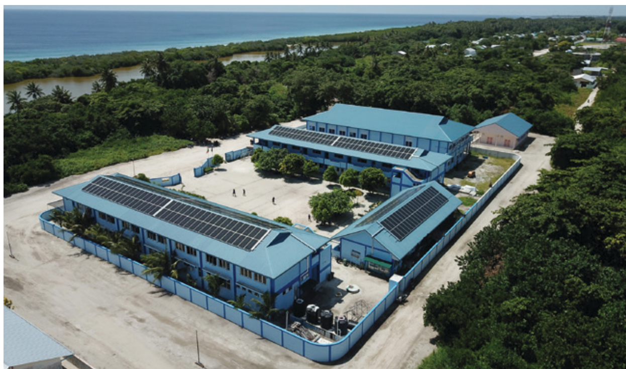
■ POISED = Preparing Outer Islands for Sustainable Energy Development Project. Solar photovoltaic panels on the roofs of schools and public buildings are connected to diesel power plants—forming hybrid systems (photo by Ministry of Environment).
