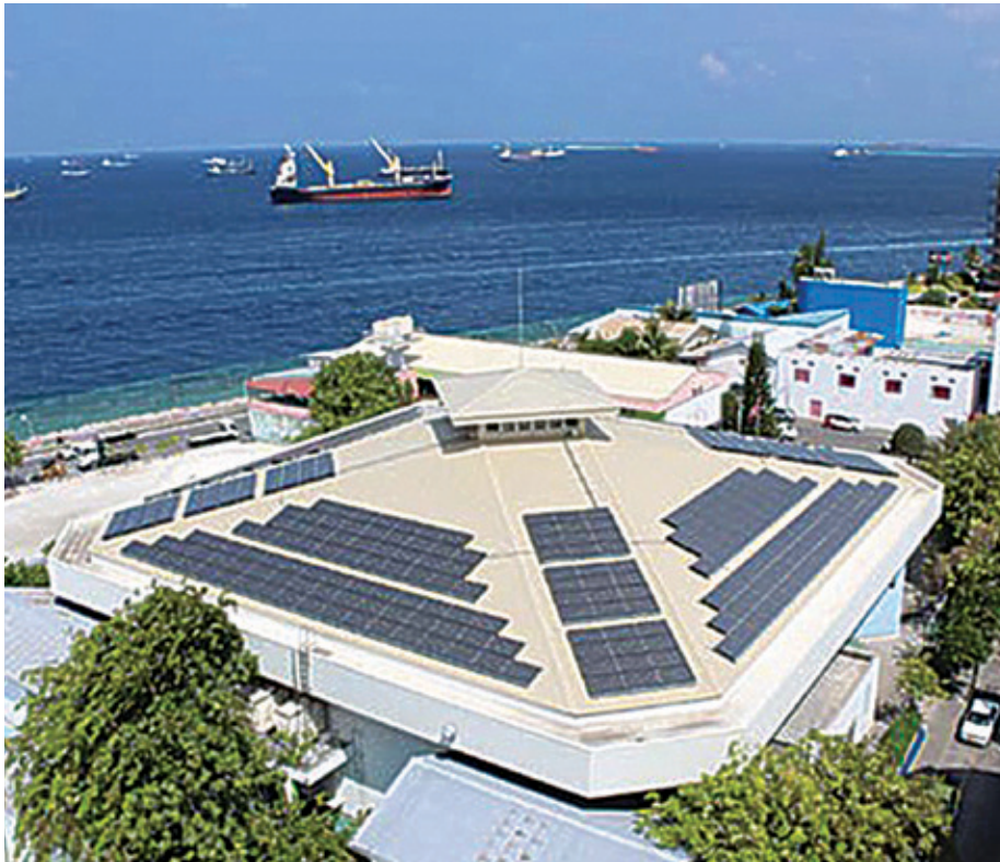
■ Rooftop Solar Photovoltaic. A 100 kilowatt-peak solar PV system was installed at Maldives Center for Social Education in Male' (photo by Ministry of Environment).
