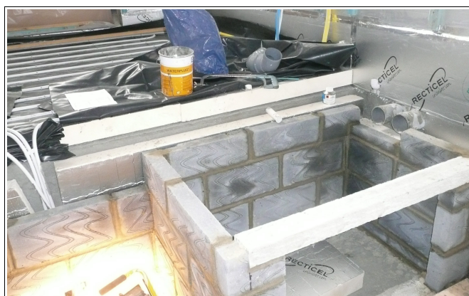
Log store under construction
