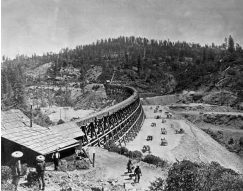
Figure 10.1 Chinese workers building the Central Pacific Railroad
