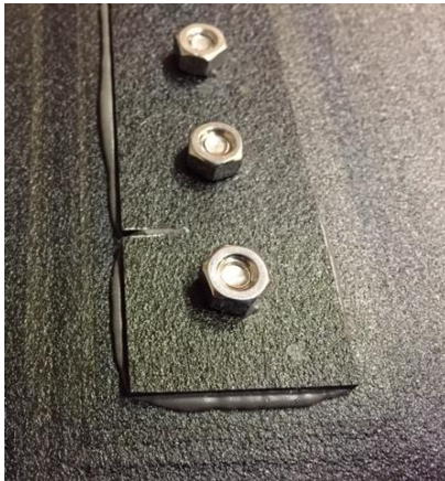
Grinder Cut *Cracked or broken substructure
