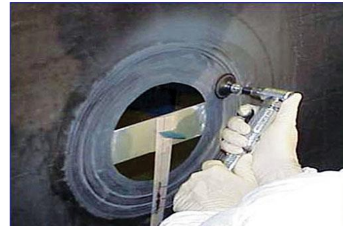
Introduction to Repairs
