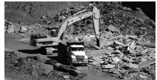
Backhoe loading truck. (Slate Valley Museum)
