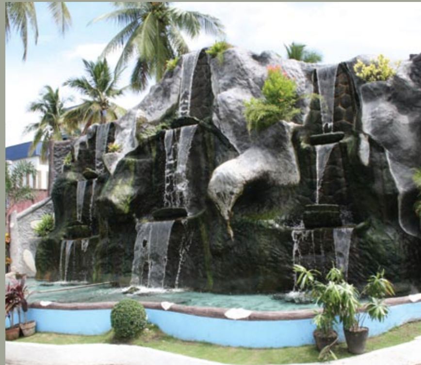
Wastewater treatment plant in CDO has been spruced up with waterfalls for a resort-like ambience
