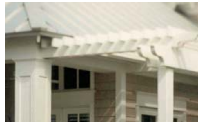
Framed lattice over more than one window.
