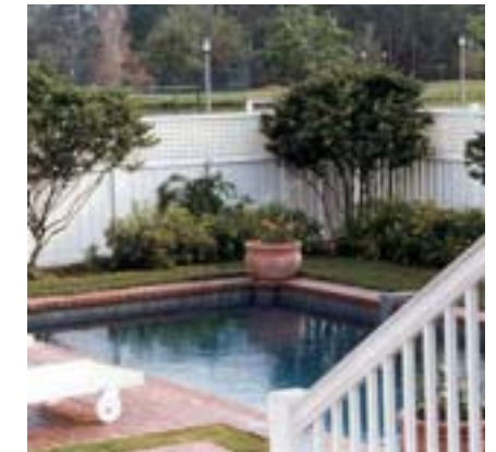
High wood fence painted white with 2/3 buttboards and 1/3 vertical lattice. See Pool Enclosures for acceptable heights.
