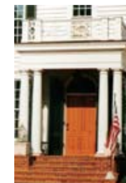
Uncovered terrace over stoop entry.
