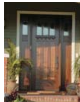
Craftsman style door with color, window grouping, paneling and hardware consistent with the historical Craftsman aesthetic.
