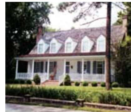
Full width additive front porch.
