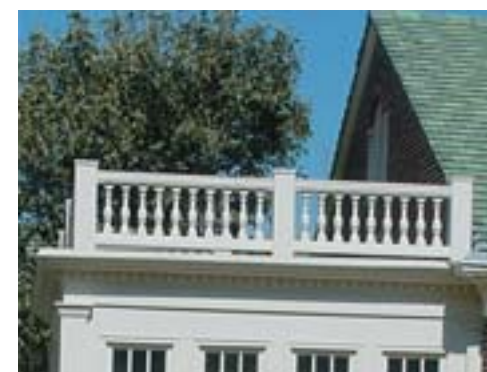
Uncovered terrace with classical guard rail detailing.
