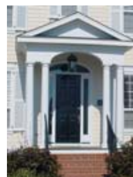
Gabled classical additive stoop porch entry.
