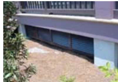
Stucco piers with louver screening.
