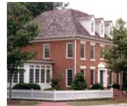
Brick veneer with stone lintels. Dormers are finished in appropriately colored lap siding.
