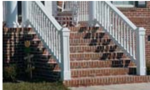
Continuous brick base with integrated brick stair.
