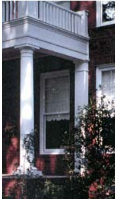
Round wood column and engaged square column with appropriate classical capital detailing and proportioning.
