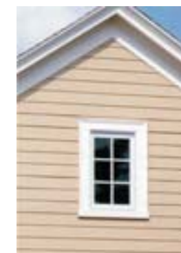
Clapboard siding and painted wood trim.
