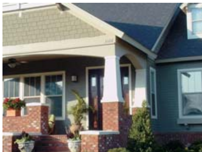
Freestanding and engaged tapered wood and brick columns. Large scale and brick base with wood or stone transition cap are consistent with Craftsman and Bungalow architectural style.
