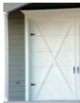
Painted wood door with cross bracing and expressed handles and hinges.
