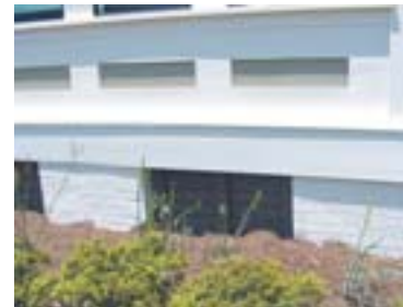
Painted brick piers with horizontal boards crawl space screening.
