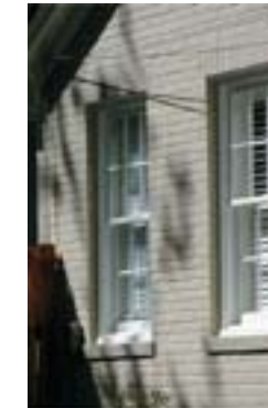
Painted brick veneer with soldier course lintel.
