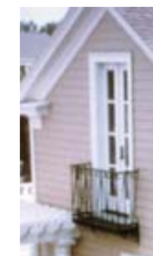
Acceptable metal balcony railing.
