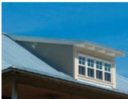
Shed dormer with exposed tapered rafters.
