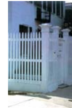
White painted picket fence with cap detailing on pickets and post.
