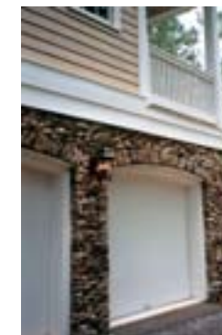
Rusticated stone base with lap siding and painted wood trim.
