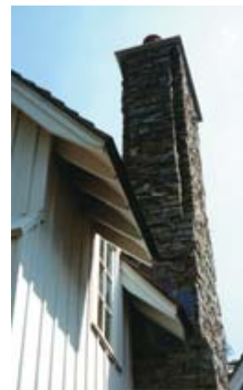
Exposed tapered rafter tails with fascia trim.
