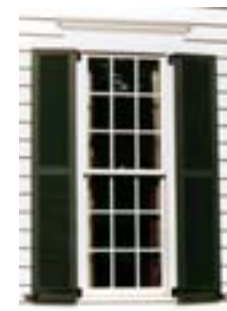
9 over 9 double hung window with classical cornice trim.
