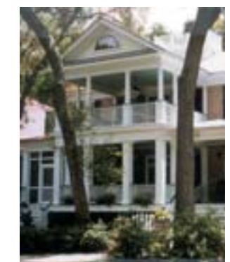
First and second level covered balconies in this double gallery porch.
