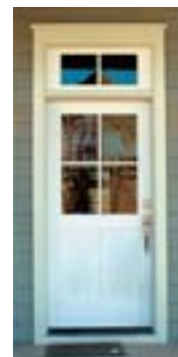
6'-8" tall door with appropriate transom, casing, and head trim.
