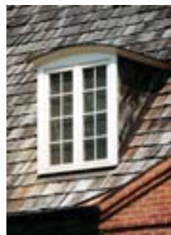
Eyebrow dormer with windows above main roof eave.
