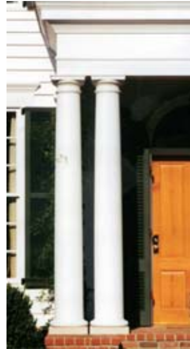
Double round columns with appropriate scale, base and capital detailing and frieze and cornice detailing.
