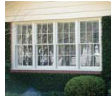
Four grouped 6 over 6 windows with appropriate trim and brick and siding surround. Groomed vine overgrowth is encouraged.
