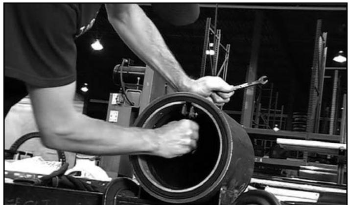
**STEP F:** Once in place, tighten the clamp to secure it against the pipe and compress the rubber adhesive strip.
