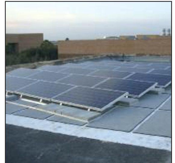
Panels on roof of Building at UTPA. (A. Pesquera)
