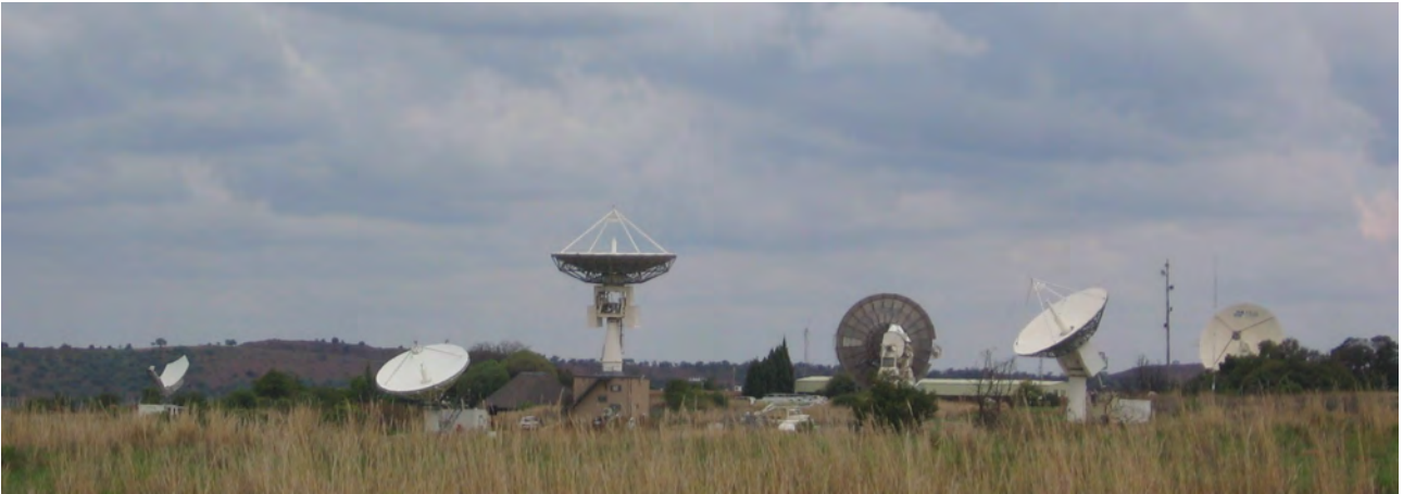
Illustration 55: The CSIR Satellite Applications Center at Hartebeeshoek near Johannesburg. Special antennae track satellites as they pass overhead and download images using radio waves.
