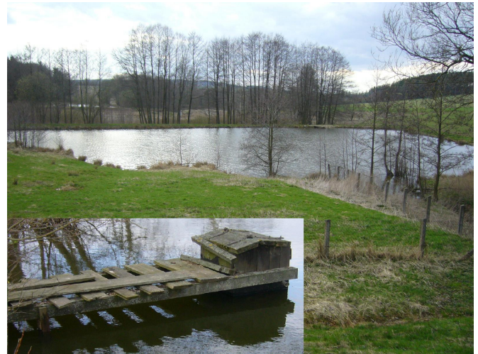
Figure 2: Small Dams: Reservoir as a part of a cascade of small dams in East Thuringia, Germany, with combined wooden Intake/Shaft Spillway (Photograph: Pohl)
